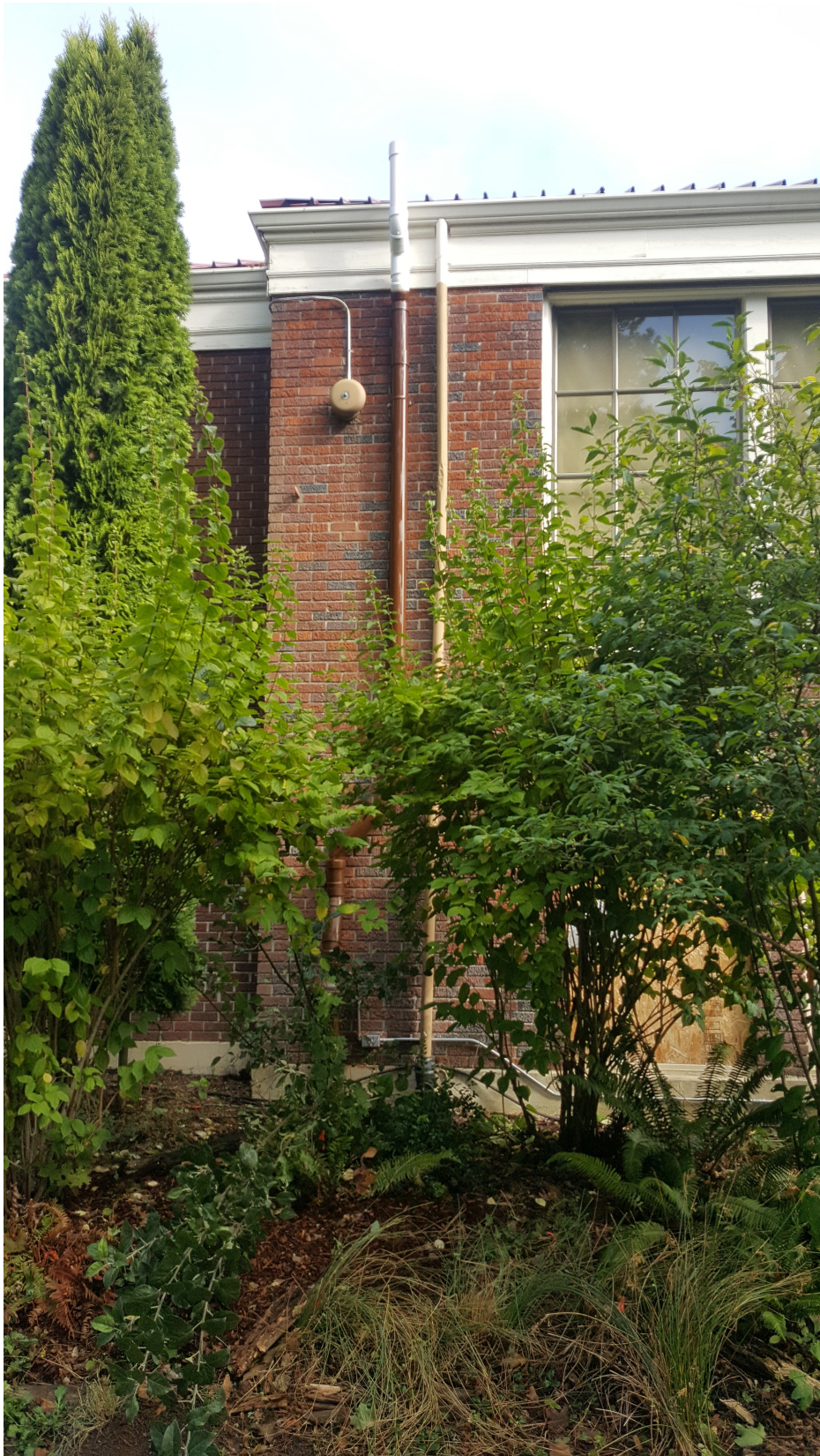
This pictures shows the fan and the continuation of the vent piping discharging above the roofline
